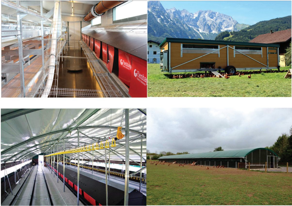
Figure 11: Indoor (left) and outdoor (right) view of a smaller multi-tier mobile house with gravity ventilation mechanically ventilated © Steiner Automation (top) and a large naturally ventilated single-tier mobile house © 2022 McGregor Structures Ltd (bottom)
