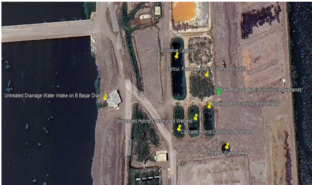
Fig. S1. Google Earth visualization of the experimental site, including the Baqar Drain, the facultative lagoon, and the 3 CWs operated in parallel.
