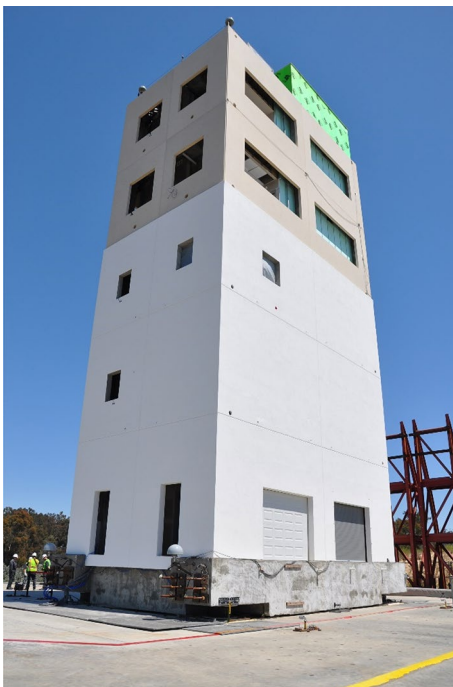
Fig. 12 Five-story RC frame building [40]
