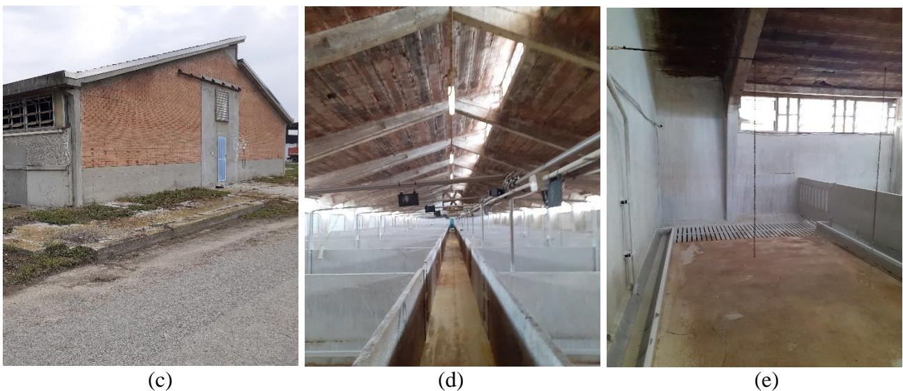
Figure 1. The case study building. (a) Aerial view; (b) Plan view of the layout; (c) External view; (d) Corridor view and (e) pen view in the wing w3.
