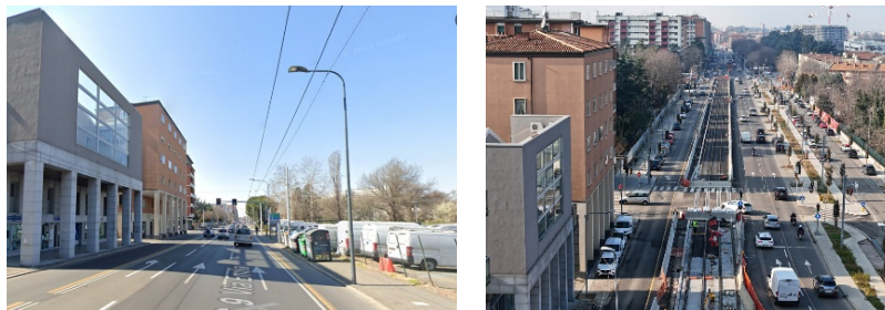
Fig.6 The west segment of the Via Emilia (Via Saffi) before the insertion of tramway's Red line (left) and then completely redesigned in its current asset with ongoing works (right)
