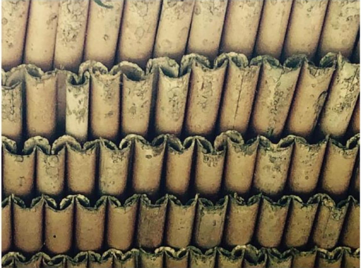
Figure 8. Simuane tallang roof detail. © Photograph: Aurora Donzelli.
