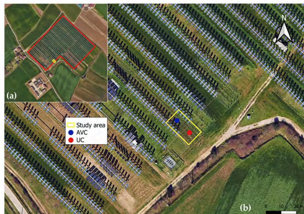
Figure 5. (b) Detailed view of the monitoring study area (yellow outline) within the agrivoltaic (AV) array, showing the location of the AVC (blue marker) and UC (red marker) monitoring plots, where volumetric water content (VWC) and soil water potential (SWP) sensors were installed at 15, 30, 45, and 60 cm depth. (a) The inset shows the position of the study area (yellow marker) within the wider AV system boundaries (red outline), as shown in Figure 1b. Imagery source: Google Earth, acquired on 12 March 2024 [29].
