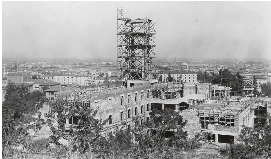
Fig. 5. Pictures of the construction phases. (historical photo: Cantieri IV - 12 © ASUB archive)
