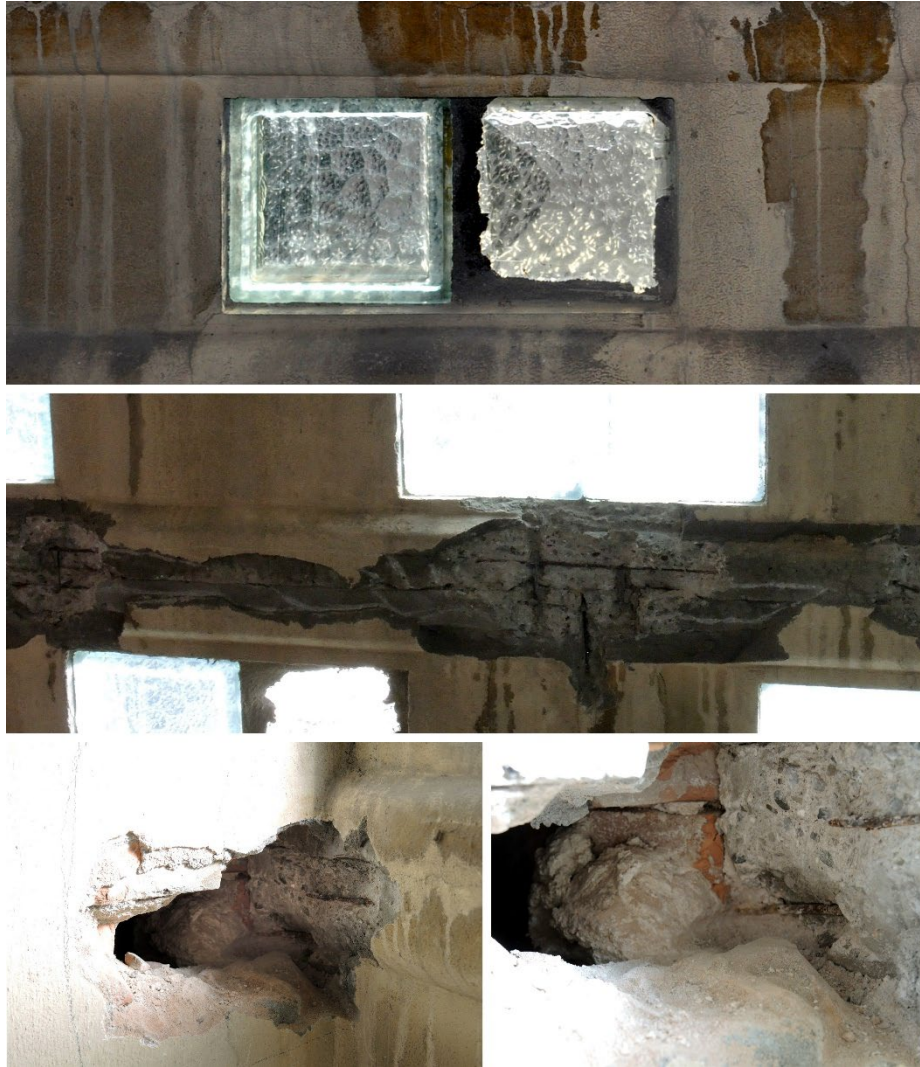
Fig. 13. Tests performed on the internal façade. (authors' original photos)
