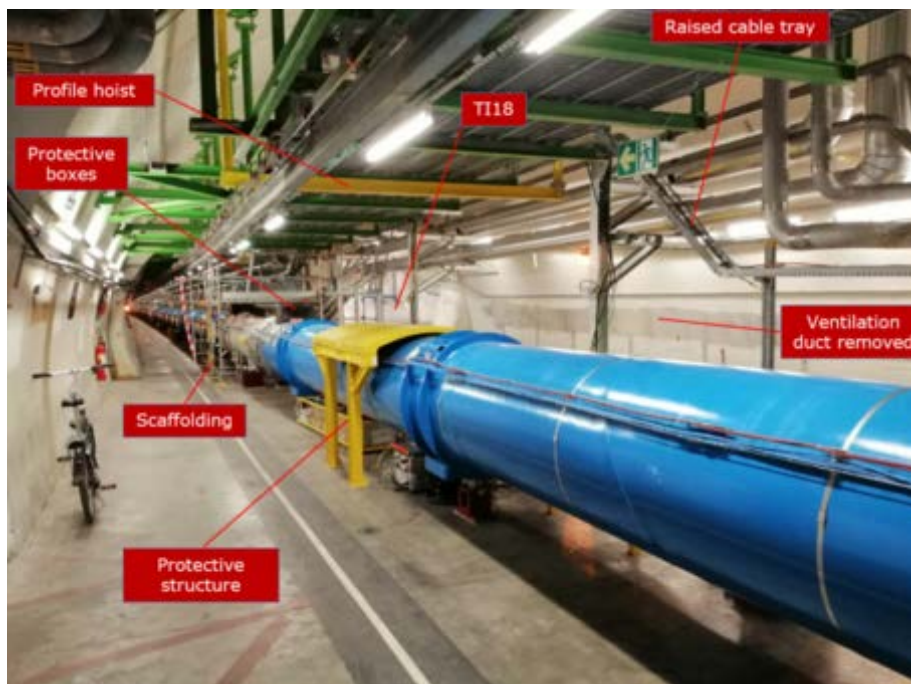
Figure 51. Principal modifications in UJ18 integration.
