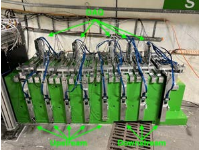
Figure 16. Picture of the hadronic calorimeter and muon system installed in TI18.
