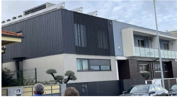
Fig. 4. View from the outside of the demonstrator building.
