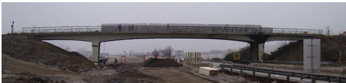
Fig. 4: View of the S101 Bridge [72].
