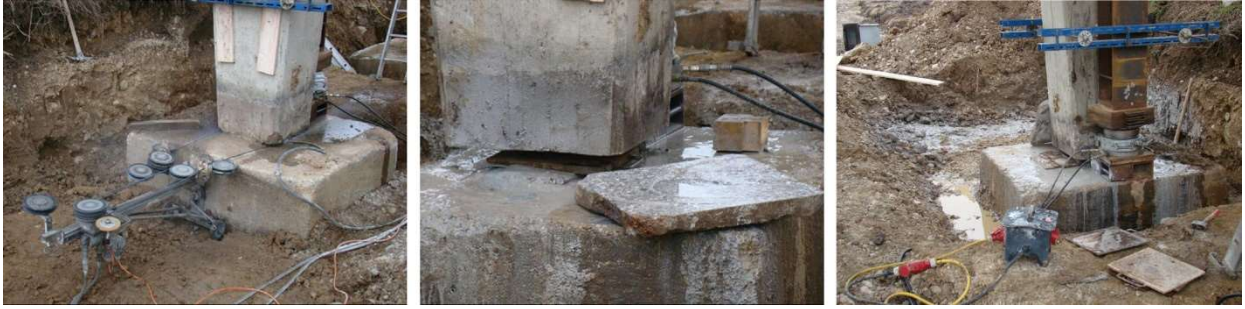
Fig. 7: Photographic documentation of the pier settlement process [72].
