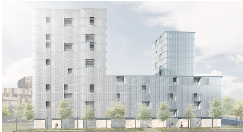
Figure 4. General view of the building articulated in differently oriented volumes for which a homogeneous façade layout was required.
