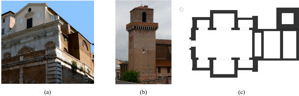
Fig. 8. San Francesco da Paola church: (a) church view, (b) bell tower view, (c) plan.
