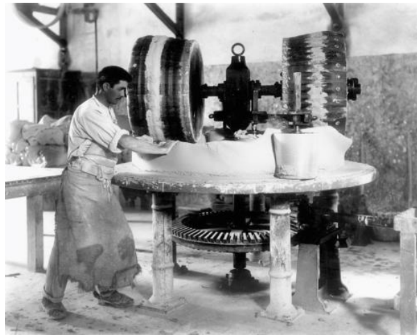
Worker at the Ginori artisan factory in Doccia (Florence) portrayed during the pressing phase of the mixture for the production of ceramics, 1902.
