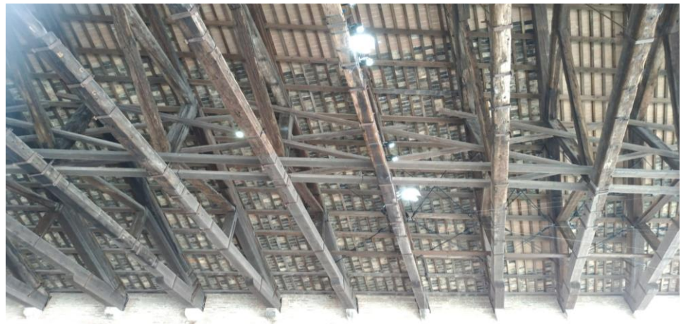
Figure 2. Bottom view of the roof.
