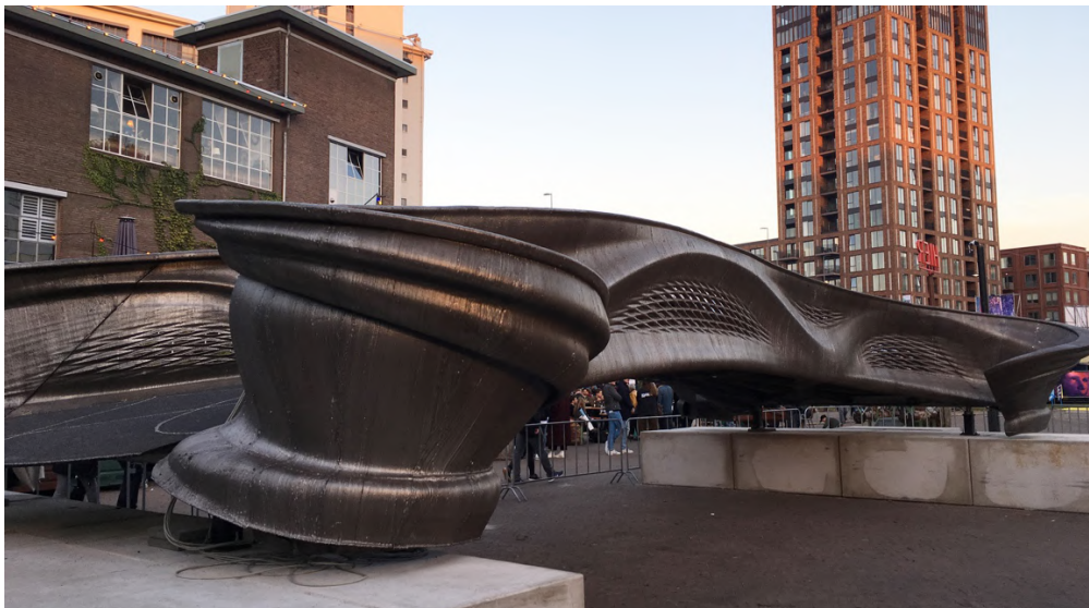
Figure 1: MX3D Bridge realized with WAAM process [16].
