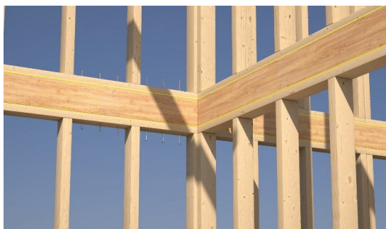
Figure 1. Example of typical structural joints with interposed acoustic layer (Rothoblaas archive).
