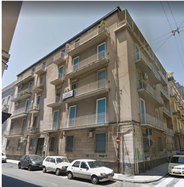
66 67 Figure 1 View of the inspiring building placed in Catania, Italy.
