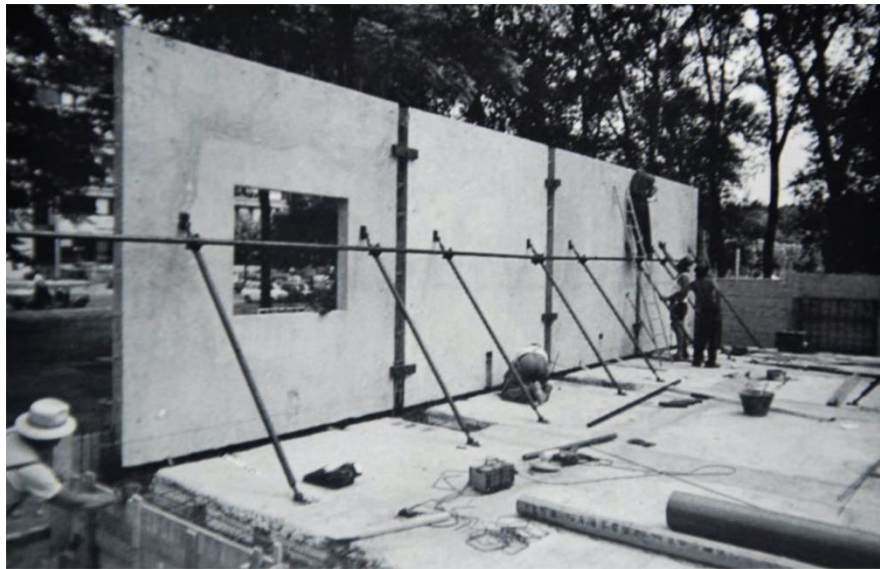
Fig. 13. Assembly of the prefabricated panels, 1977 (courtesy of G. Gresleri's Archive)
