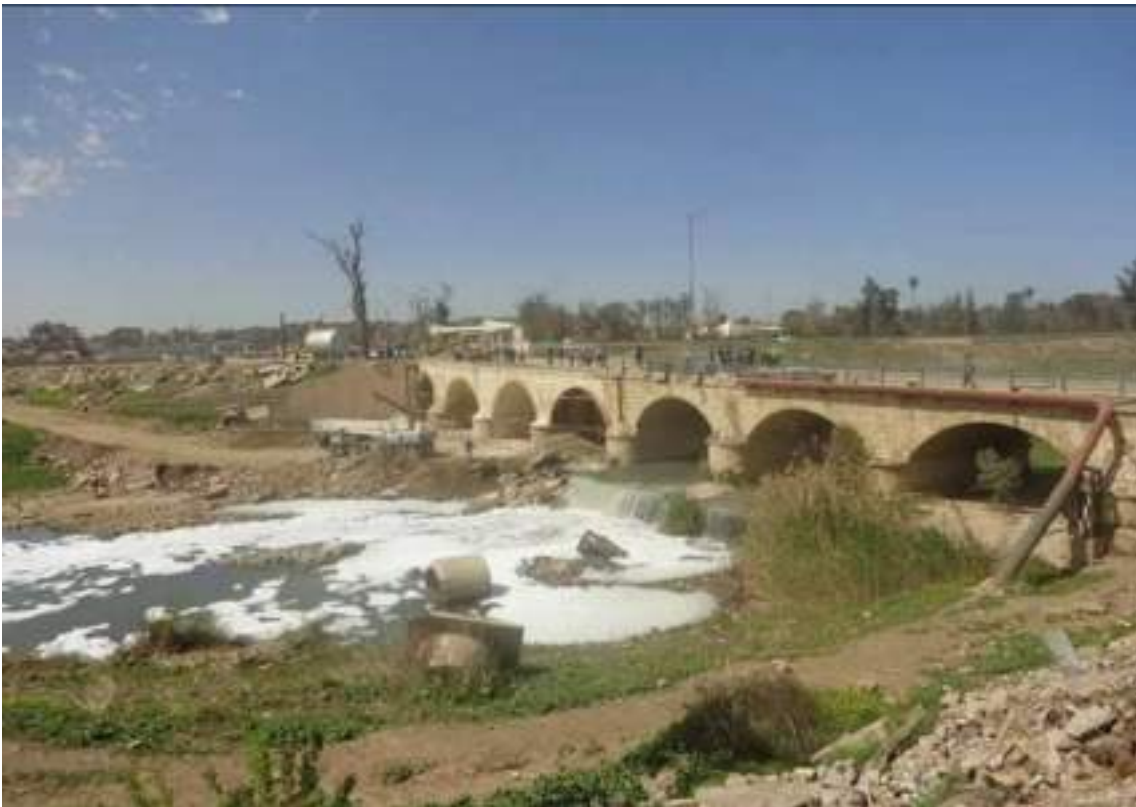
2. West end of lower Khosr bridge. View from east, after 2016, Google Maps.
