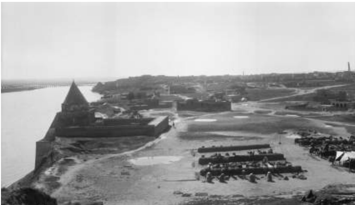
2. Distant view of Old Bridge before installation of New Bridge. Imam Yahya on left, with British cavalry(?) horses feeding. View from north-west, 1919-1920. Photograph N. 3658, probably taken by James Henry Breasted. ISAC Institute for the Study of Ancient Cultures, University of Chicago.
