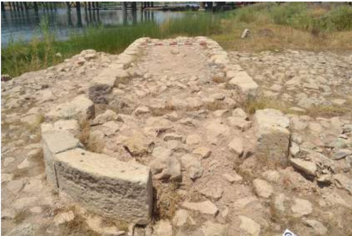
1. Pier 1 from south-east.
