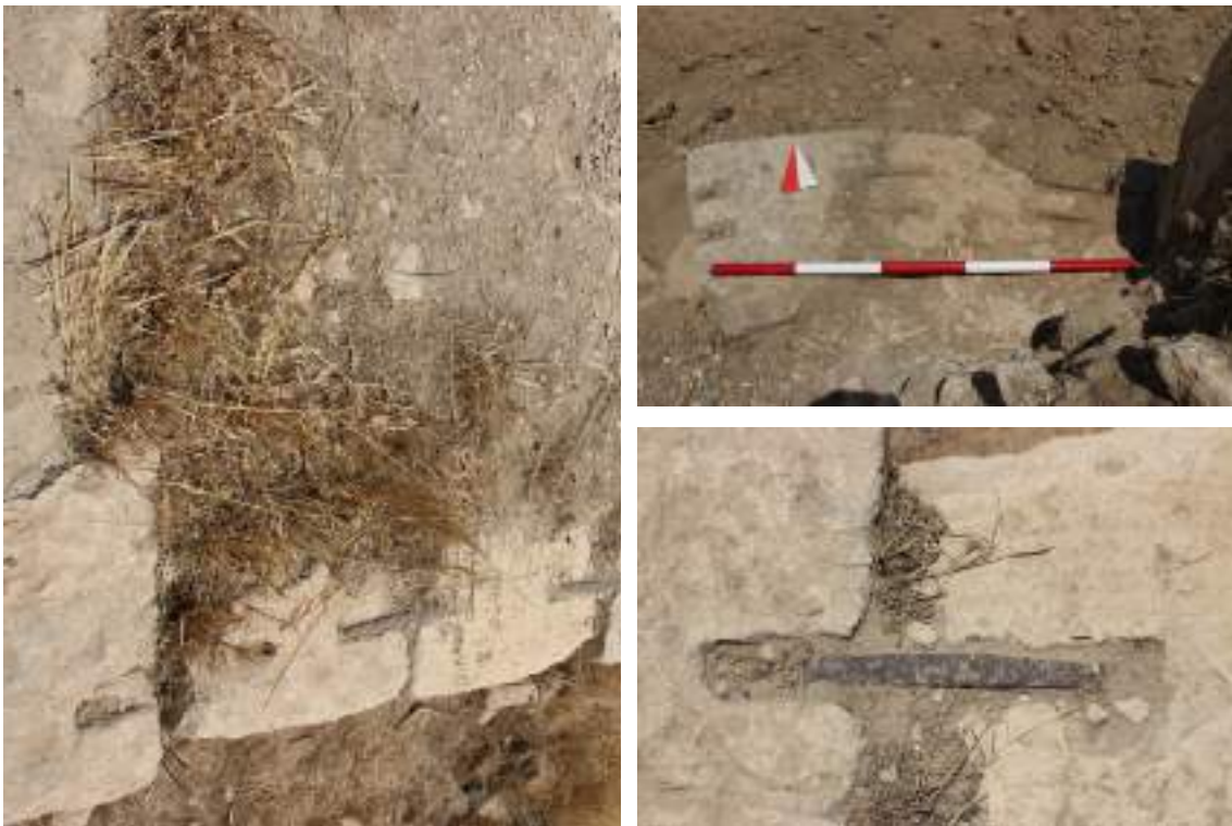
1. Iron clamps interlocked the blocks from the second course upwards. Left: sequence of grooves for the clamps in the upper face of the south-western side of Pier 3; right (above): pair of parallel grooves lodging iron clamps; right (below): iron clamp.
