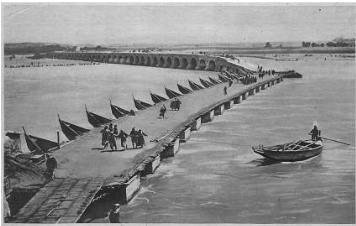
2. Pontoon bridge and Old Bridge. Views from south-west: Pontoons in position, after rebuilding of ramp, c. 1906-1914. Photographer unknown.
