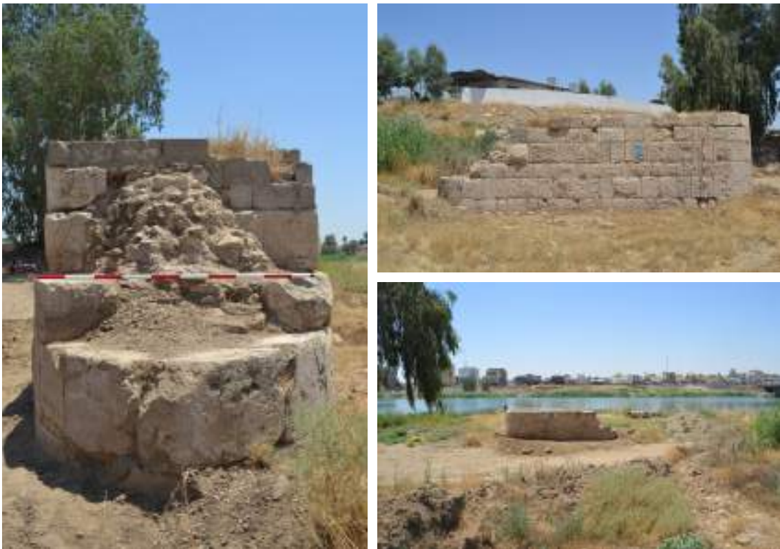
1. Pier 3. Left: view from north-west; right (above): view from west; right (below): view from east.
