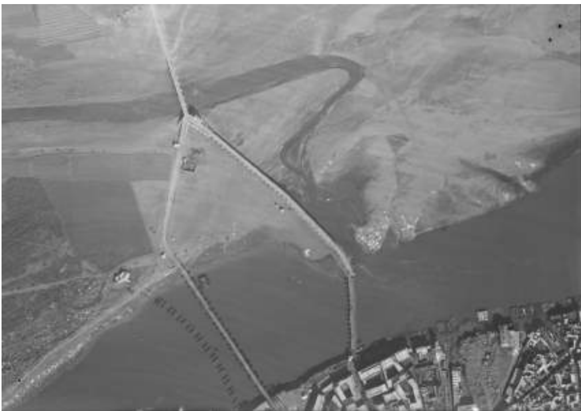
2. Bridges across Tigris and Khosr. From left to right: breakwater, New Bridge and Old Bridge, with lower Khosr bridge at top. Detail from R.A.F. photograph, A.P.610, c. 1920s. University College London.
