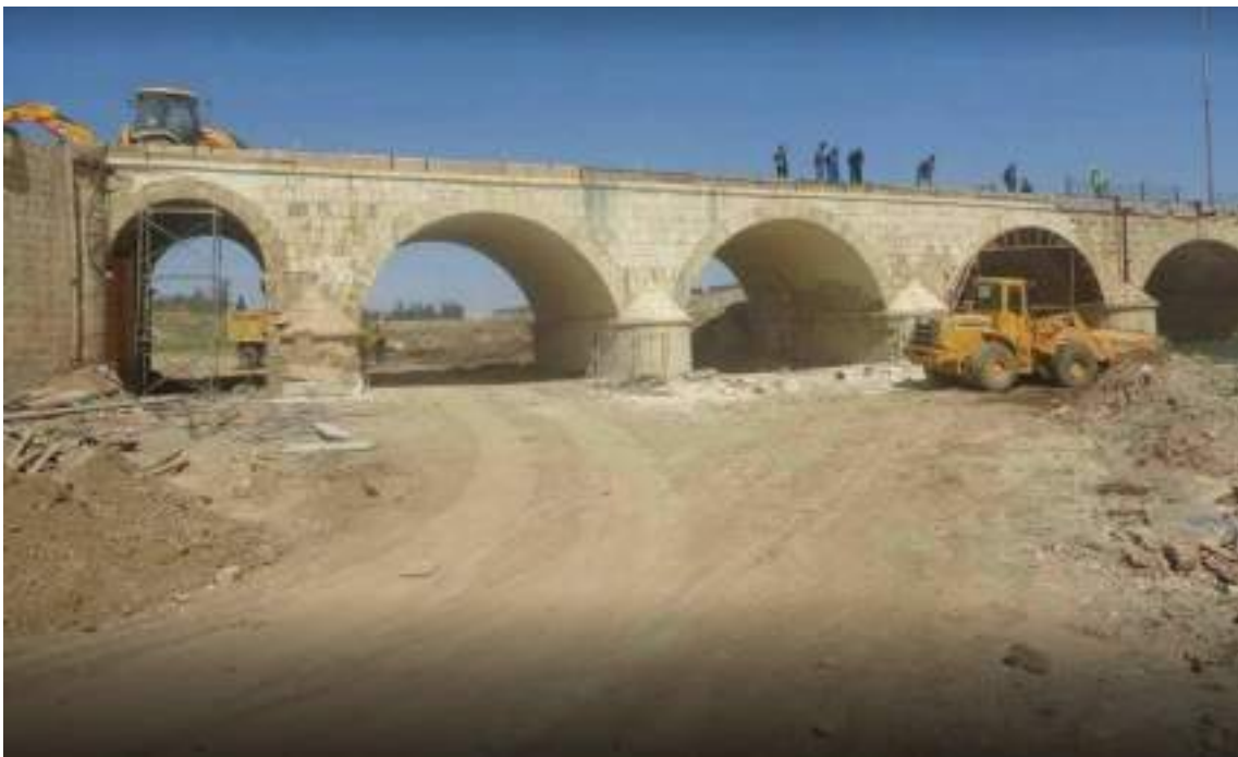
2. East end of lower Khosr bridge under repair. View from south, c. 2019. Image by Adnan Adnane, 2020, Google Maps.
