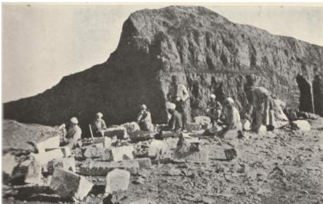
2. Workmen removing stone from wall of Nineveh between Kuyunjik and Nabi Yunus, c. 1919. Budge 1920: II, fig. facing p. 6.
