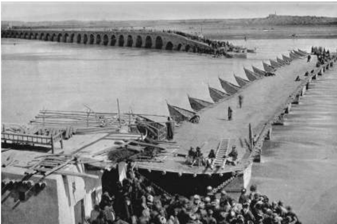
1. Pontoon bridge and Old Bridge. Views from south-west: Pontoons being hauled into position, 1905-1908. Hume-Griffith 1909: fig. facing p. 176
