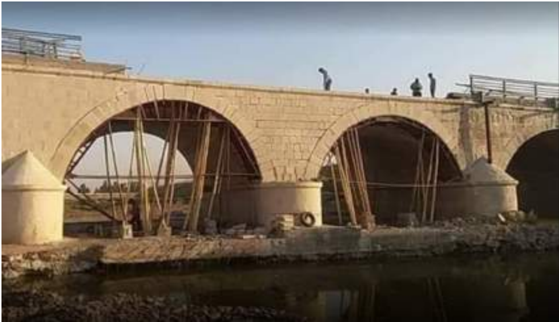
1. Centre of lower Khosr bridge under repair. View from south, c. 2019. Image by Aamir Fadel, 2020, Google Maps.
