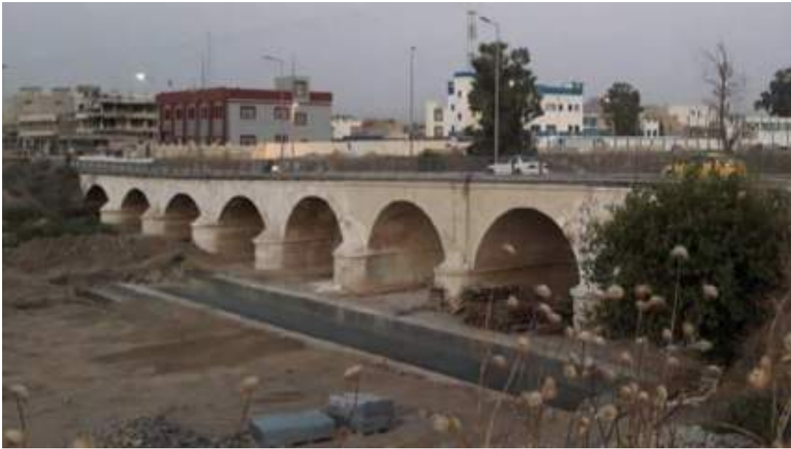
1. North side of lower Khosr bridge. View from west, c. 2022, Google Maps.
