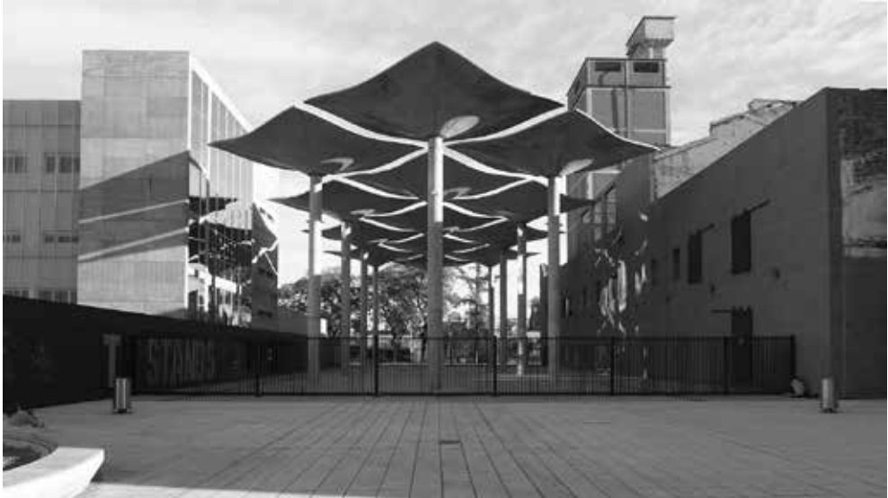
III. 2. Roofing of a collective space in a public square in Santa Fe (El Molino, Fábrica Cultural, 2010) in Argentina, photo: Gino Malacarne.
