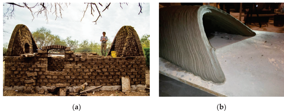
Figure 4. The Nubian vault: (a) Traditional Nubian vault construction technique using raw earth bricks [27]; (b) Prototype of a vault 3D-printed with 40^\circ inclined layers without supports [28].
