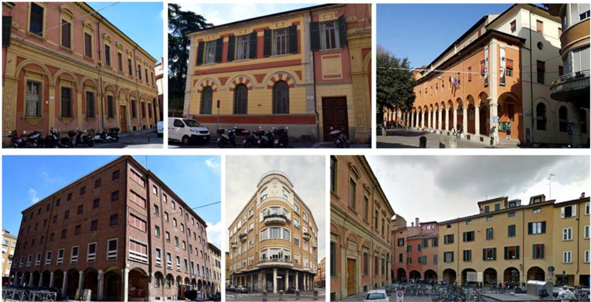
Figure 2. (From left to right, first line: university library, department of economics, national gallery of Bologna and fine arts academy; second line: university student house and canteen, sundial building and ancient residential buildings © Predari)
