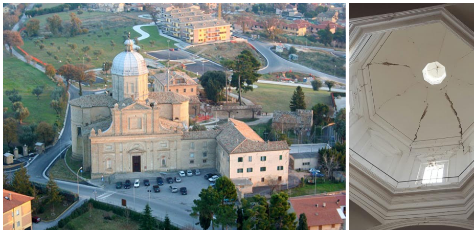
Fig. 1. - Aerial photo of the church of Santa Maria delle Vergini in Macerata before the 2016 earthquake (on the left) and the dome damaged in 2016 (on the right).
