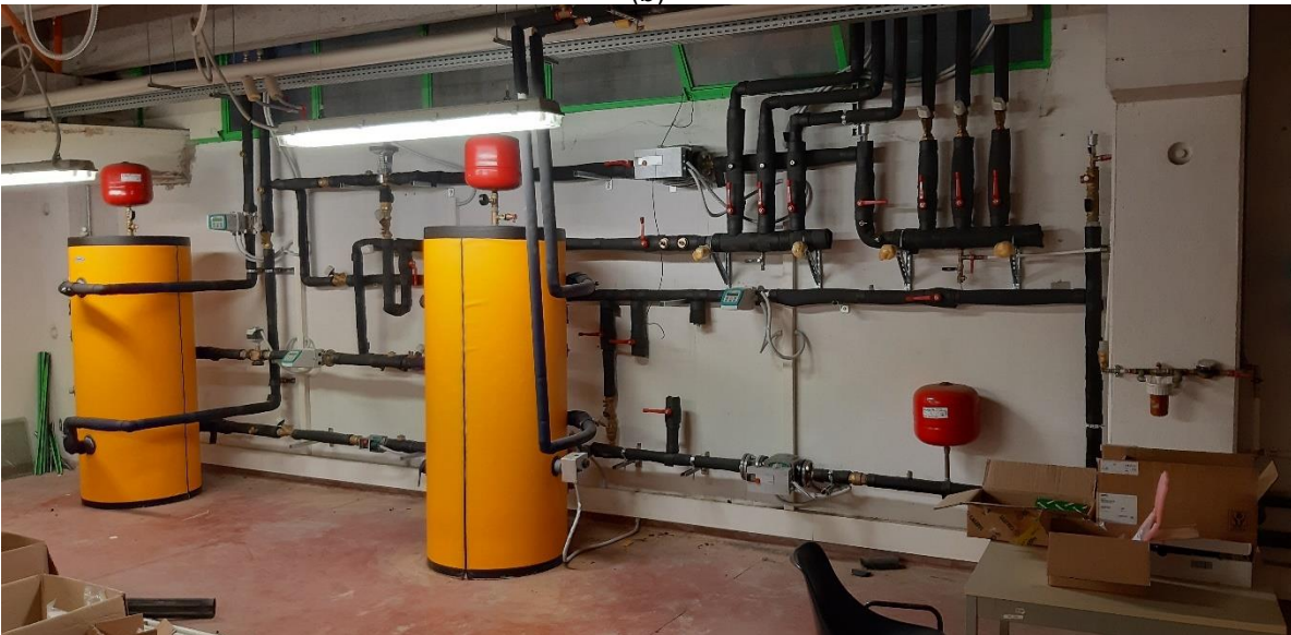
230 Figure 3. Air-heaters inside the climatic chamber (a) and the hydronic loop of the test rig 231 (b).
