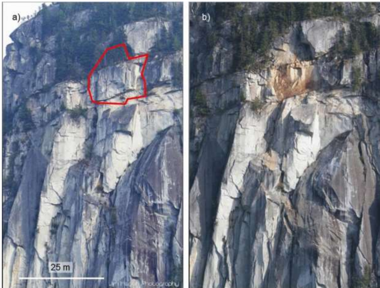
Fig. 6 Pre- and post-failure photographs of a rockfall failure in Squamish, B.C., Canada (Golder Associates, 2015 in Sampaleanu 2017)
