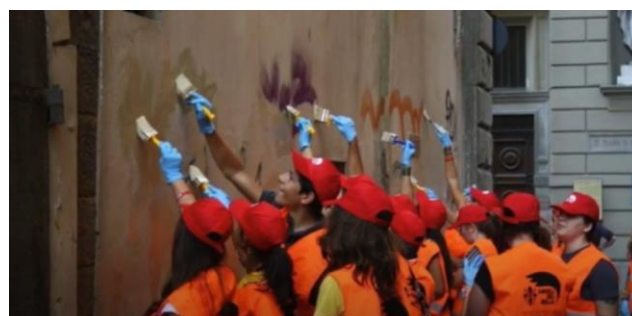
Figure 4 – Cleaning of walls of the historical centre
