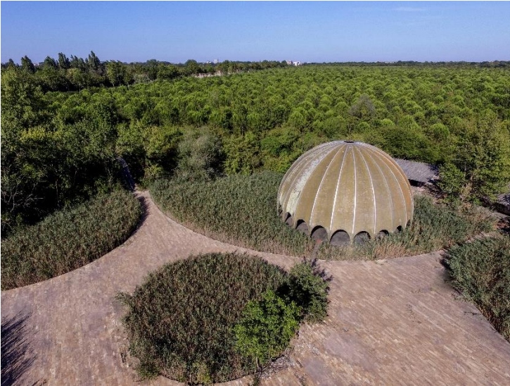
Fig. 3 Current state of the Woodpecker dance club, invaded by vegetation (the photo was taken through the drone described in § 3.1).
