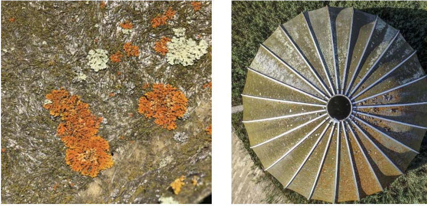
Fig. 10 Lichens on the external surface of the dome. On the left: emerging mat and differences between lichens. On the right: north-oriented zenith view of the dome, where lichens of different colours depending on the orientation can be seen (the photo was taken through the drone described in § 3.1).
