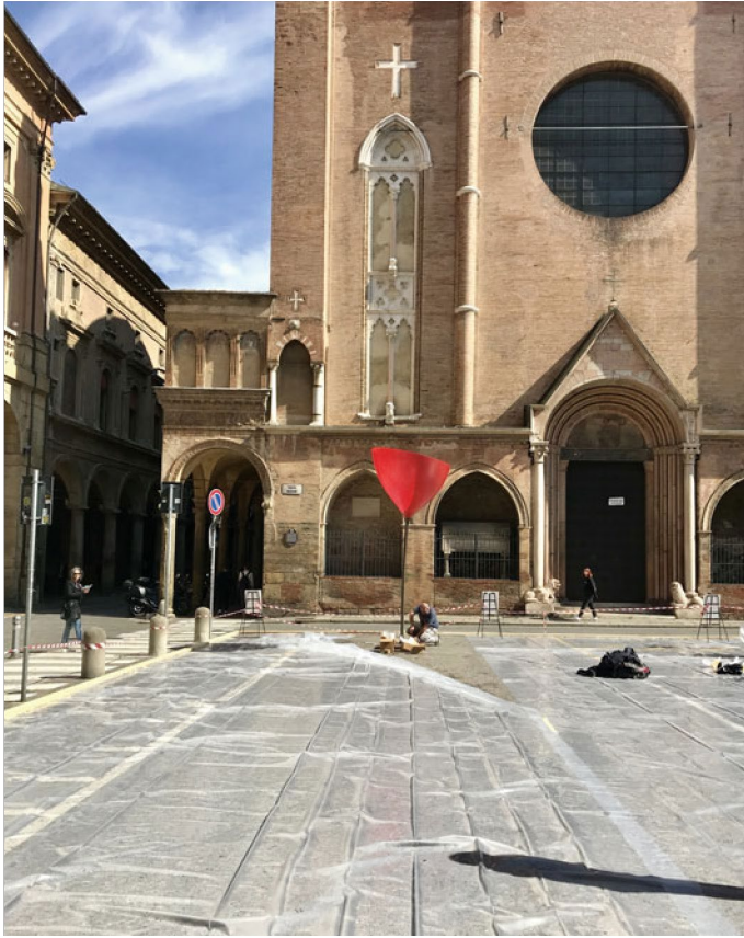
Fig. 5 Self-construction workshop reportage. Day one: safe delimitation of the area and coverage of the asphalt paving with a plastic sheet
