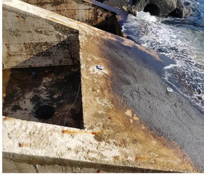
Fig. 7. Pressure transducers installed on the OBREC device.
