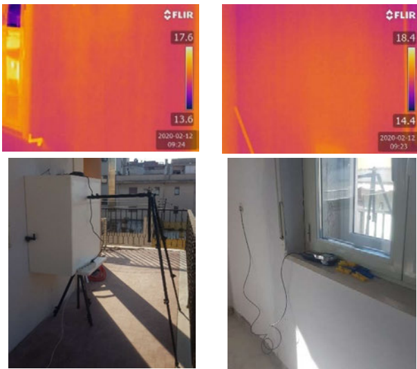
Fig. 2. Thermographic analysis and instruments installed for one of the case studies
