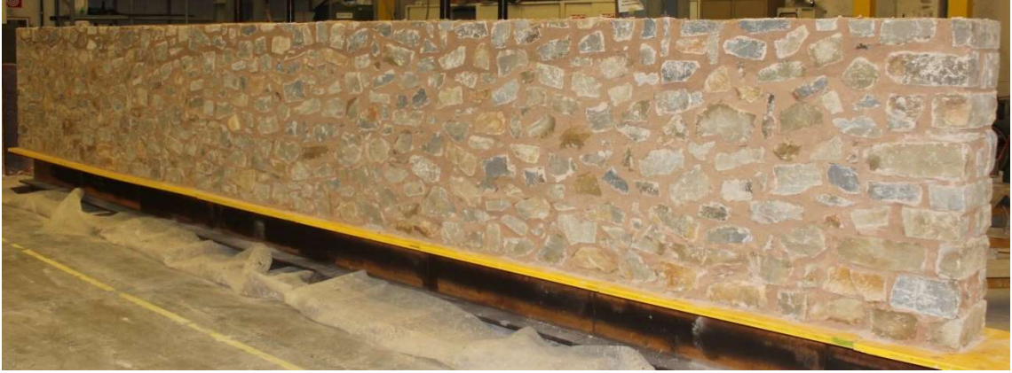
Figure 1. Stone masonry wall.
