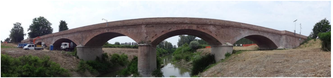
4 5 6 7 8 9 10 11 12 13 Figure 2 The test site: “Motta di Cavezzo” bridge (Modena, Italy). 14
