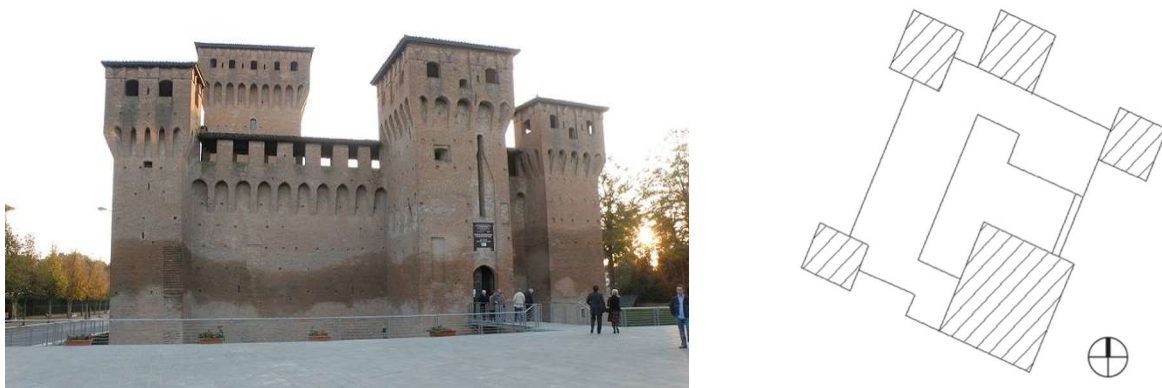
Fig. 3 - North façade of San Felice sul Panaro Fortress (view before the Emilia earthquake, 2012) and schematic floor plan.
