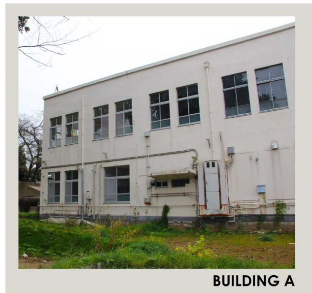
Figure 3: Building case of study (A).
