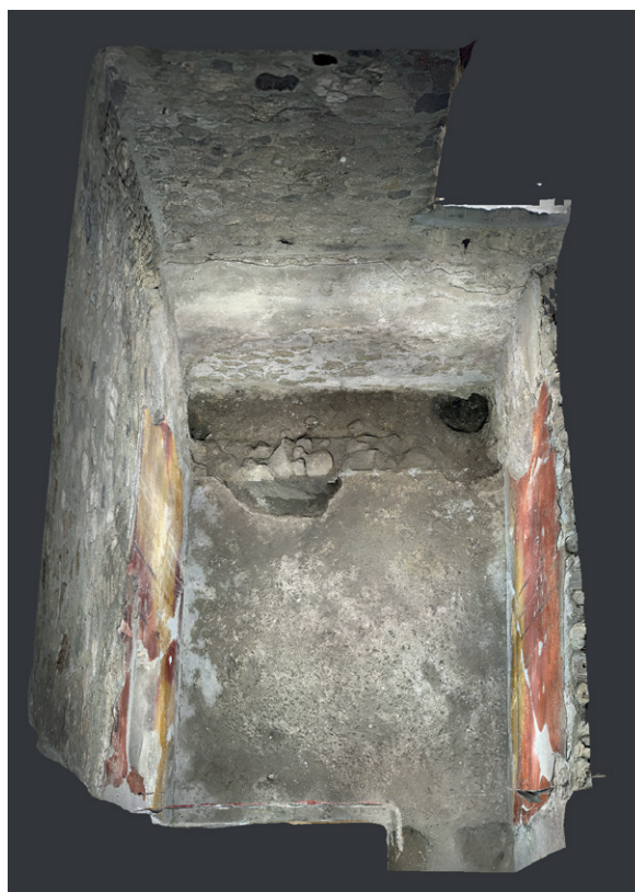
Fig. 5. Pompeii, I 17, 4. Casa degli Archi, room 3, trench F: on the east side, along the boundary wall of the insula, the demolished and razed wall (Vesuviana Programme, Pompeii Project -, F. Filippov, 2023).
