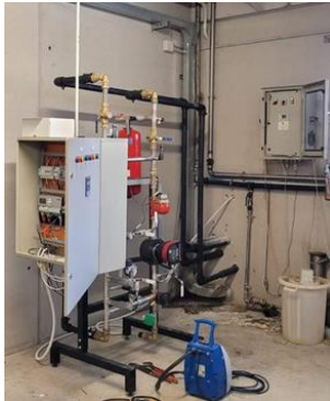
Figure 5: Standardized Solar Central Station
