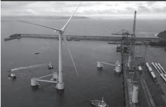
Installation & Tow-out to Site – Port of Ferrol WTF installed at quayside and towed fully assembled to site
