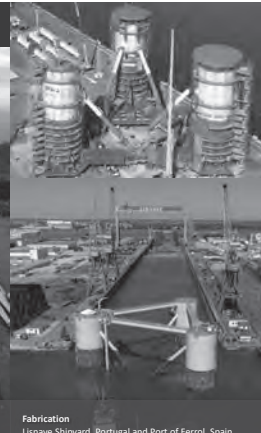
Fabrication Lisboa Shipyard, Portugal and Port of Ferrol, Spain
