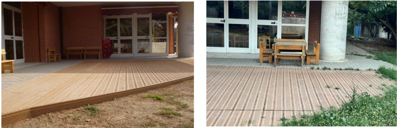
Fig. 10 An emblematic WPC project: a kindergarten outdoor decking in 2008, as built, and in 2024
