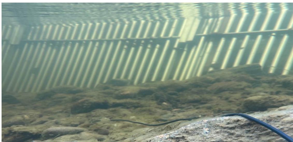
Figure 14 Underwater recording of the rattling sound from the trap-fence system installed in Deanušaldi to prevent pink salmon ( Oncorhynchus gorbuscha ) from migrating up the Deatnu (Renzi 2023).
