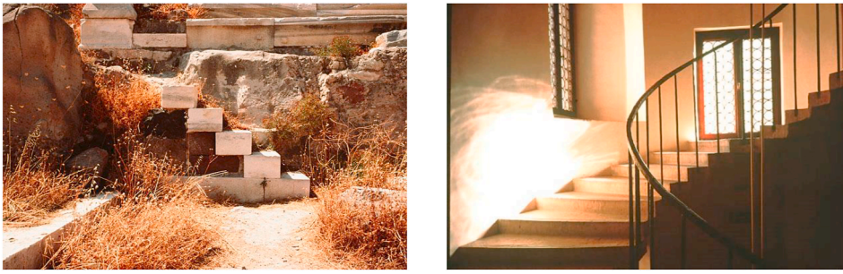
Fig. 1. Stone cantilever stairs. Left: example of straight unrebrated treads found in Milos, Greece. Right: example of spiral Palladio's stair at the Academia in Venice, Italy.
